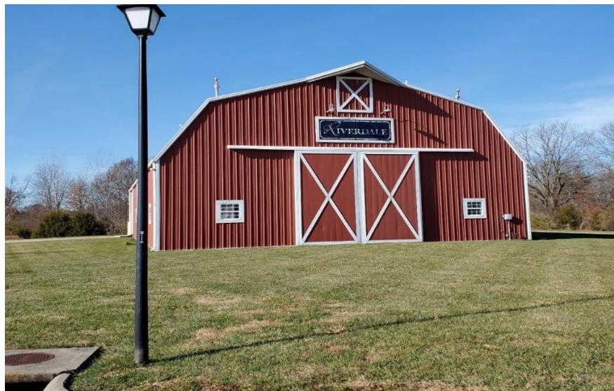
MBR sewage plant located within the adjoining Riverdale Subdivision
